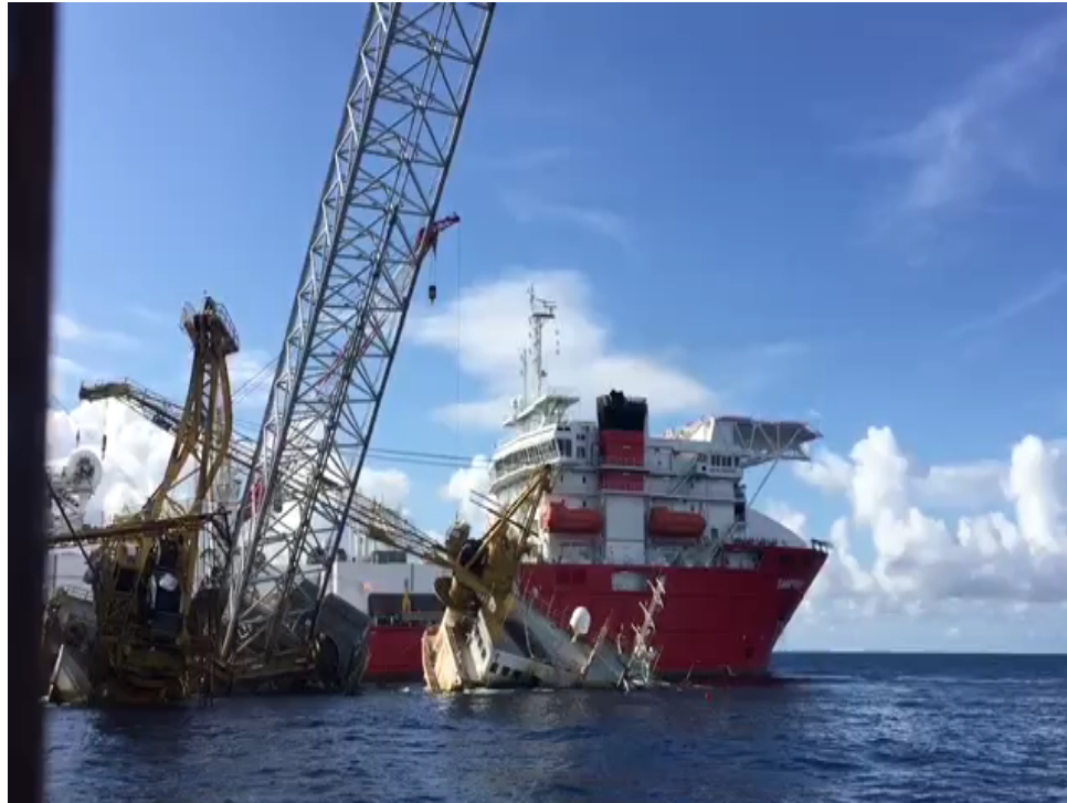
Cutting of upper port leg
